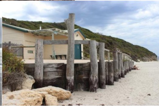
Figure 2.13 Erosion Event at Ocean Beach Timber Retaining Wall Pre (SE top June 2016) During (August 2016) and Recovered (March 2017)
