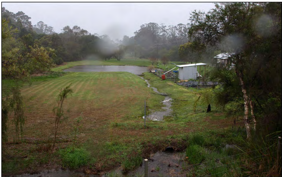
Figure 6: View east for Option 2, here the road will require a dam to be in filled and will require a large area of land to be raised in height for the connecting road to Scotsdale Road. Past the dam the alignment swings to the south east to cross the river
