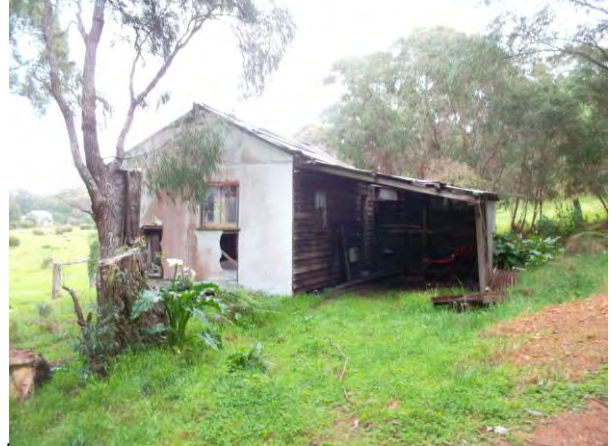
Photograph 2 – View of old shed in north west of Subject Site.
