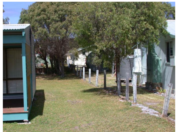
Photo 56 Simple dressed posts with mesh or wire infill have little visual impact
