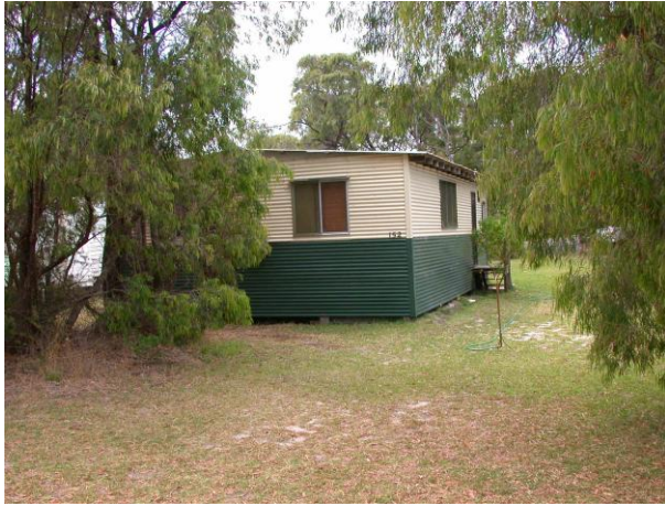
Photo 19 Authentic cladding has been replaced with colorbonded corrugated steel
