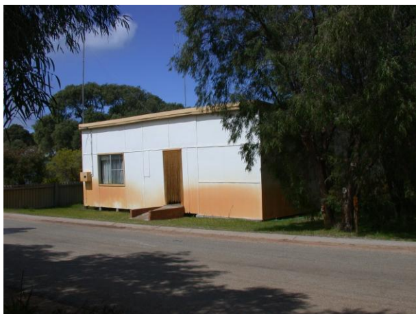
Photo 13 Typical fibro skillion in authentic condition
