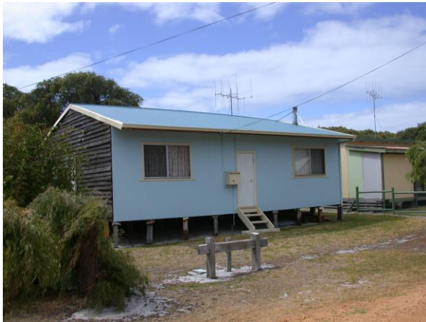
Photo 23 The timber boarding to the front of this cottage has been replaced with flat cement sheet
