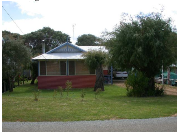
Photo 24 House has recently been extended and reclad with corrugated customorb
