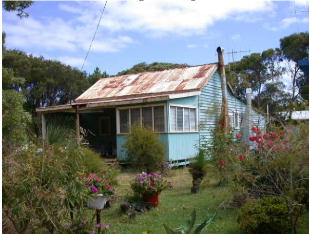
Photo 5 Jarrah clad mill cottage
