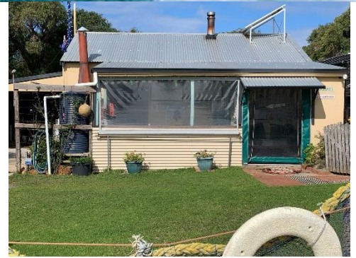
Figure 6: The current caretaker's cottage at Parry Beach
