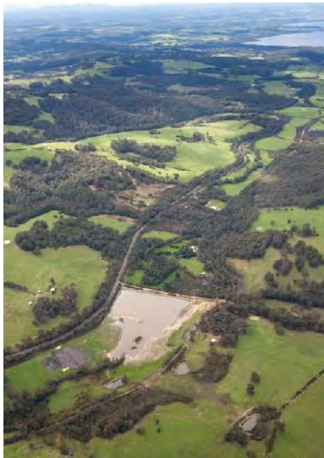
Figure 3: Aerial photo of the site looking east towards Denmark town
