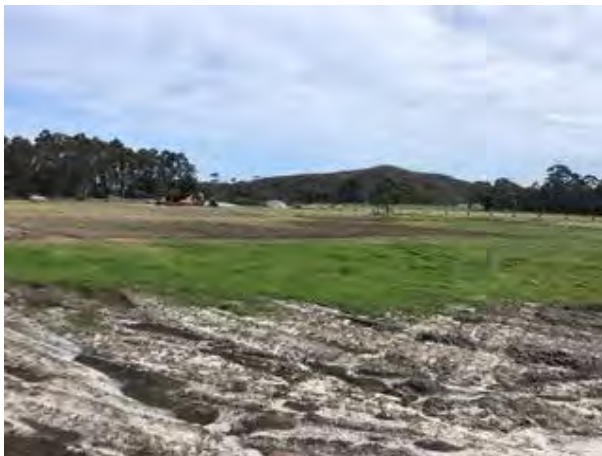
Figure 5: Bottom of dam looking SW
