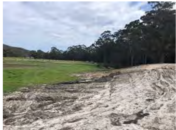
Figure 6: Bottom of dam looking W
