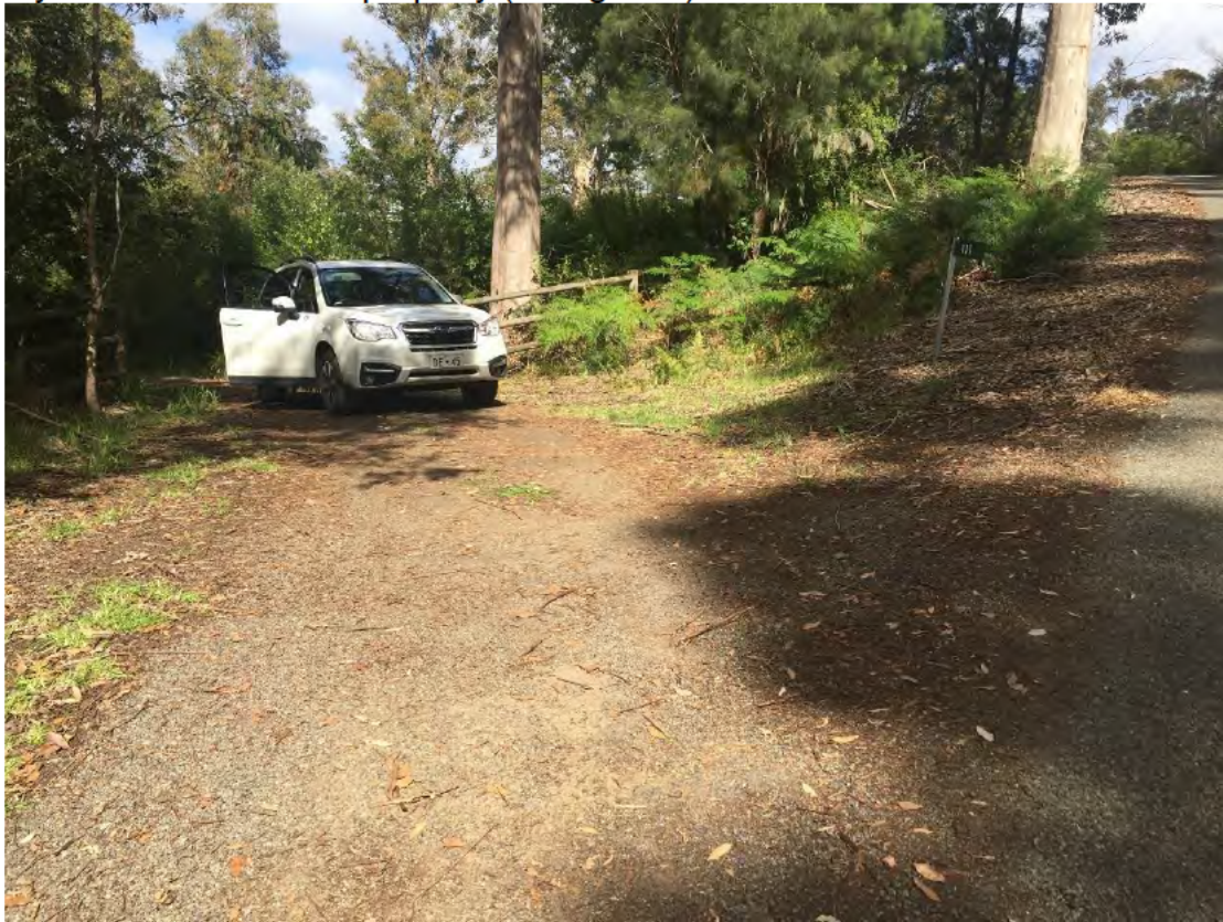
Existing crossover (Bitumen seal beneath gravel)
