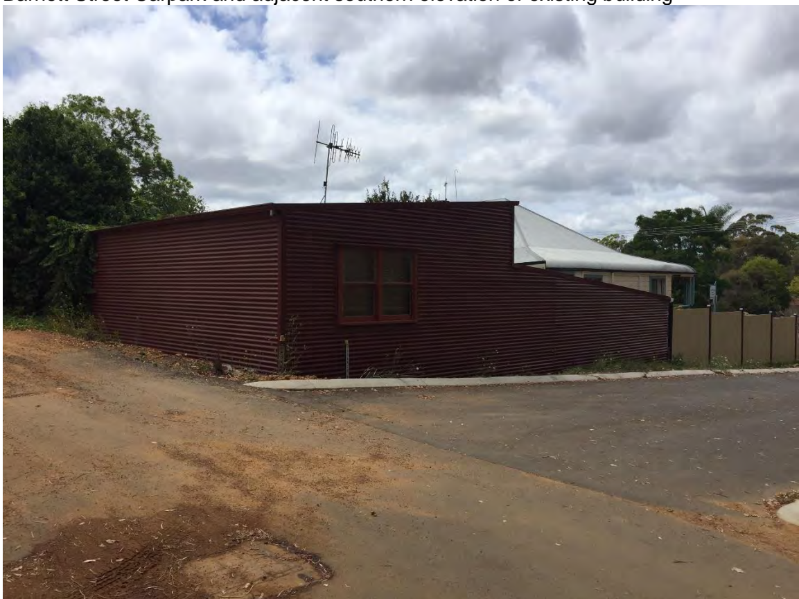
View of existing building at junction of Praed Lane and Barnett Street (carpark)
