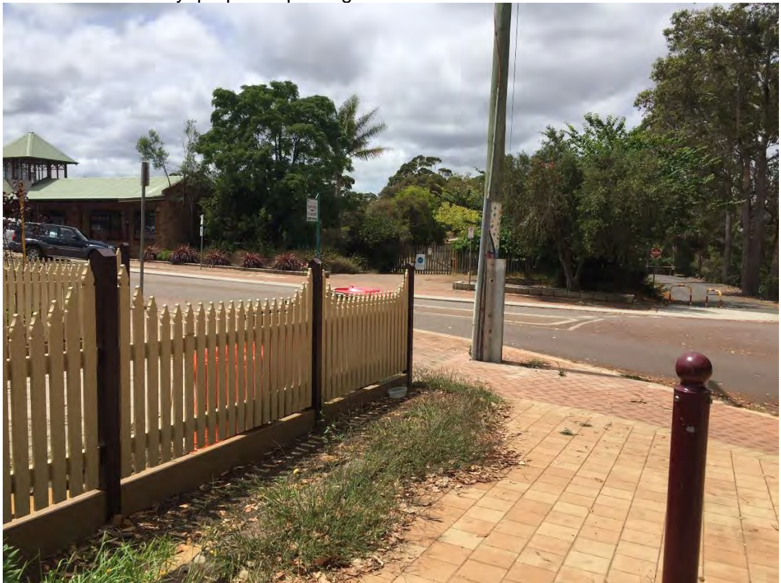
Existing fencing and power pole in proximity to driveway
