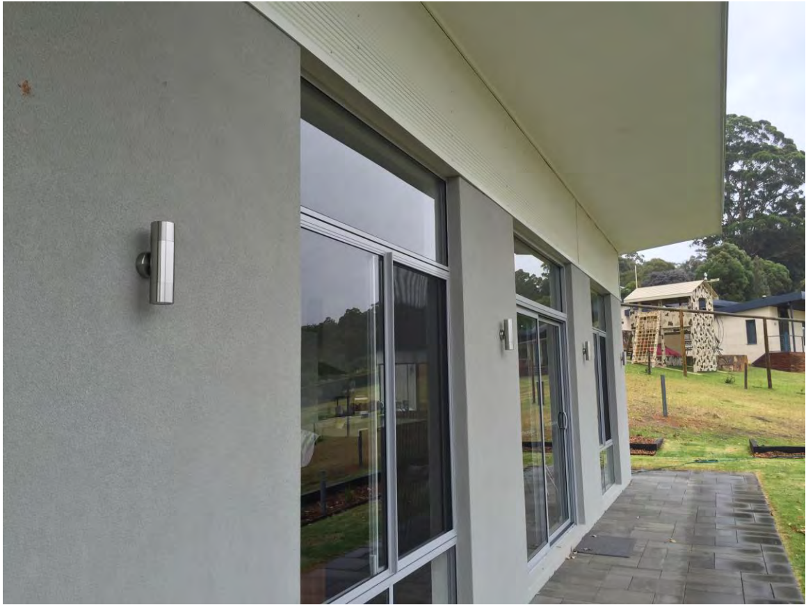
Lights on rear elevation –wall and eaves.
