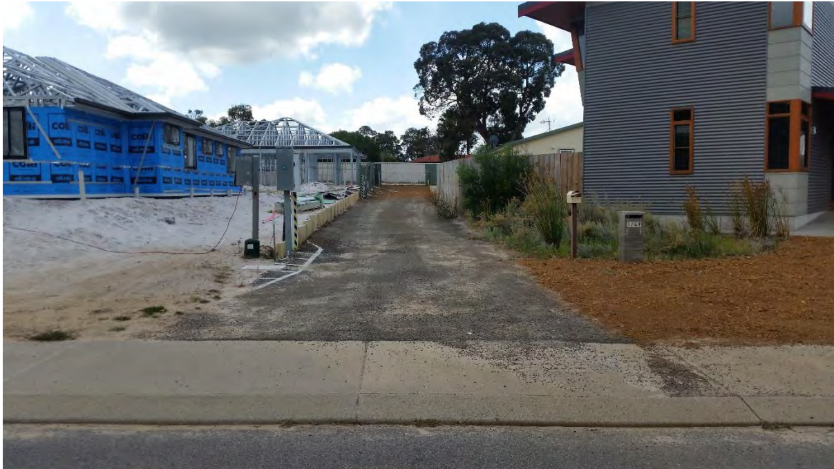
Common property driveway sealed with bitumen tack coat.
