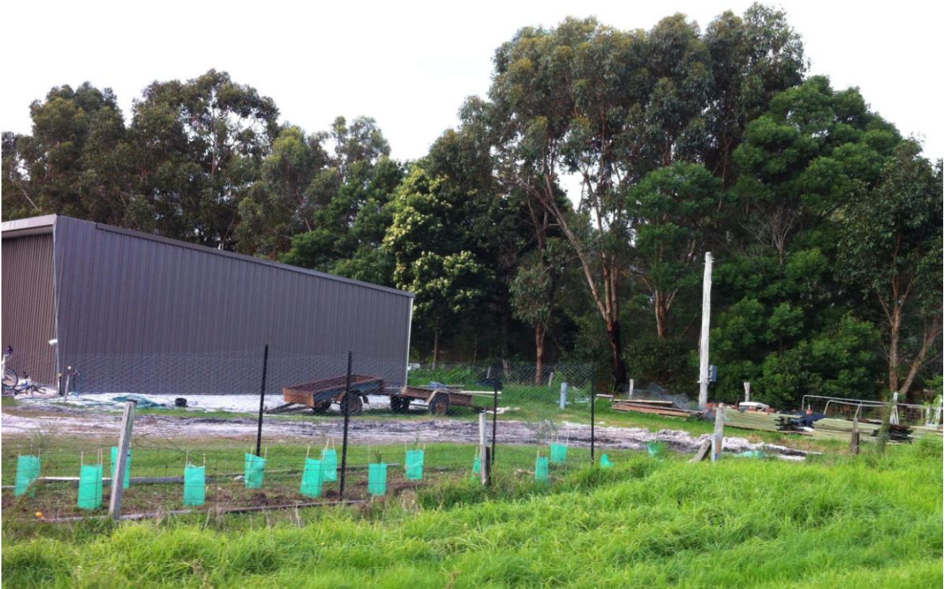
Figure 2: From street towards Outbuilding, rainwater tanks would be located adjacent this elevation
