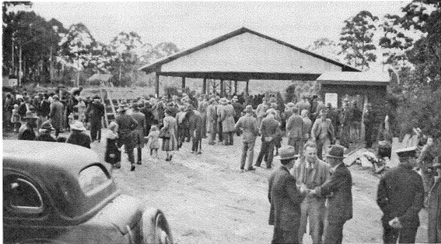
Sheds and yards at the No. 3 Railway Station site.
