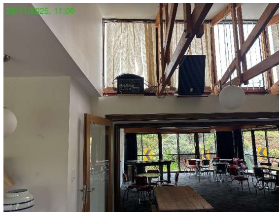
Photo 13.15.1 North light windows were not inspected in detail, but they aluminium domestic type and aged.
