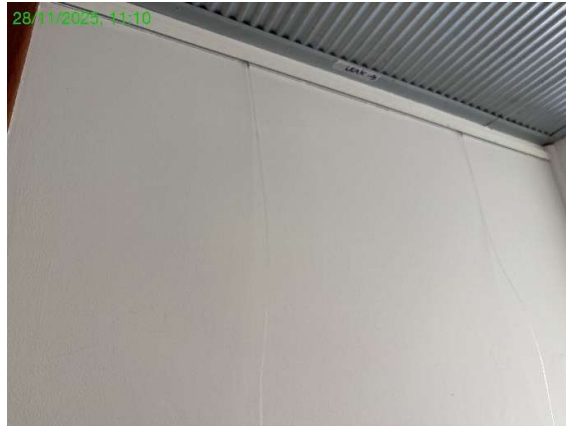
Photo 13.14.1 Photo is typical of water dripping down passage walls throughout the length of the passage.
