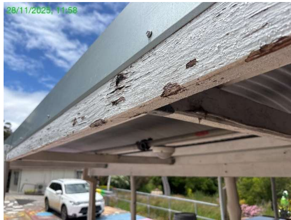
Photo 13.21.1 Entry beam with timber rot.
