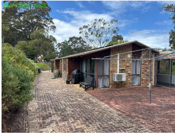
Photo 13.3.1 Note DP directly behind the R/hoist to be connected to the sump to the right/middle of C/yard.
