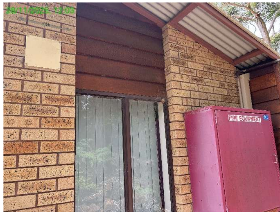
Photo 13.7.1 External Fire Hose Reel Cabinet (paint required)
