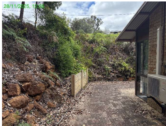
Photo: 13.4.1 No safety fence at top of embankment.
