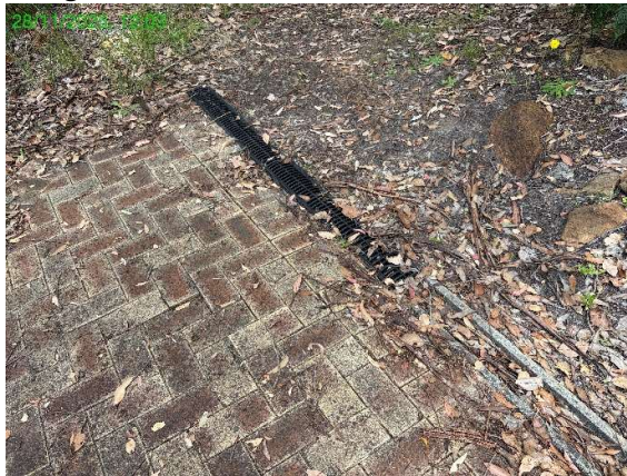
Photo 13.6.1 Grate and spoon drain to be maintained.
