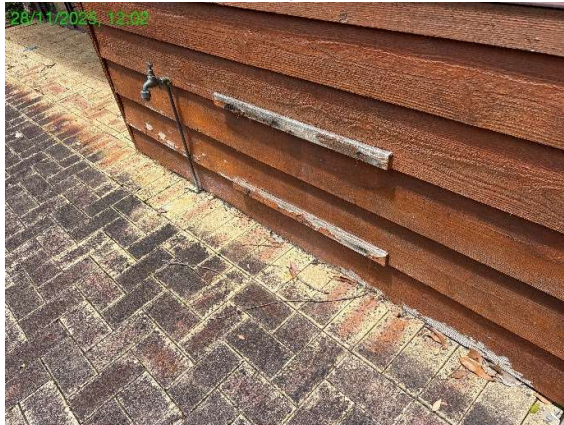
Photo 13.6.1 Discoloured paving.
