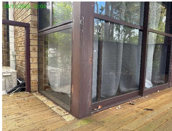
Photo 13.15.1 Aluminium cover rivets have failed on several windows.
