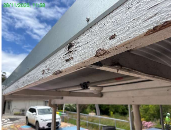
Photo 13.6.1 Timber rot and metal balustrade in the background.
