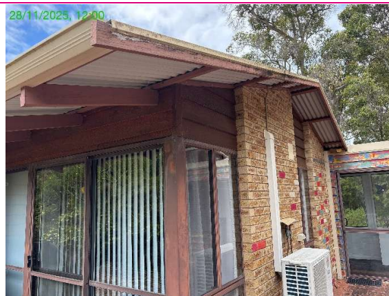
Photo 13.20.1 Paint fascia board and seal tails.
