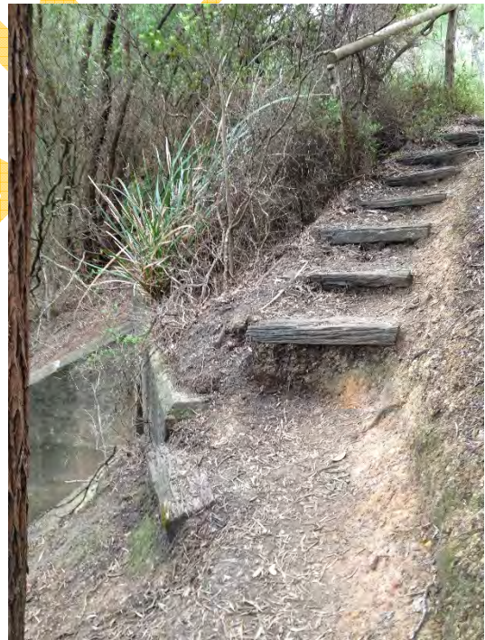
Plate 12 Access to the Springdale Tunnel to the south of the Heritage Trail requires upgrade of steps and handrail
