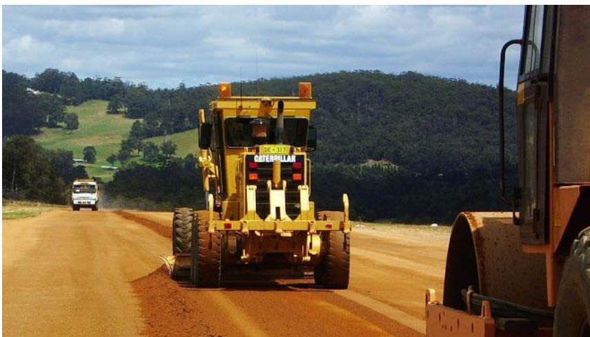
Preparations for paving runway 2010.
