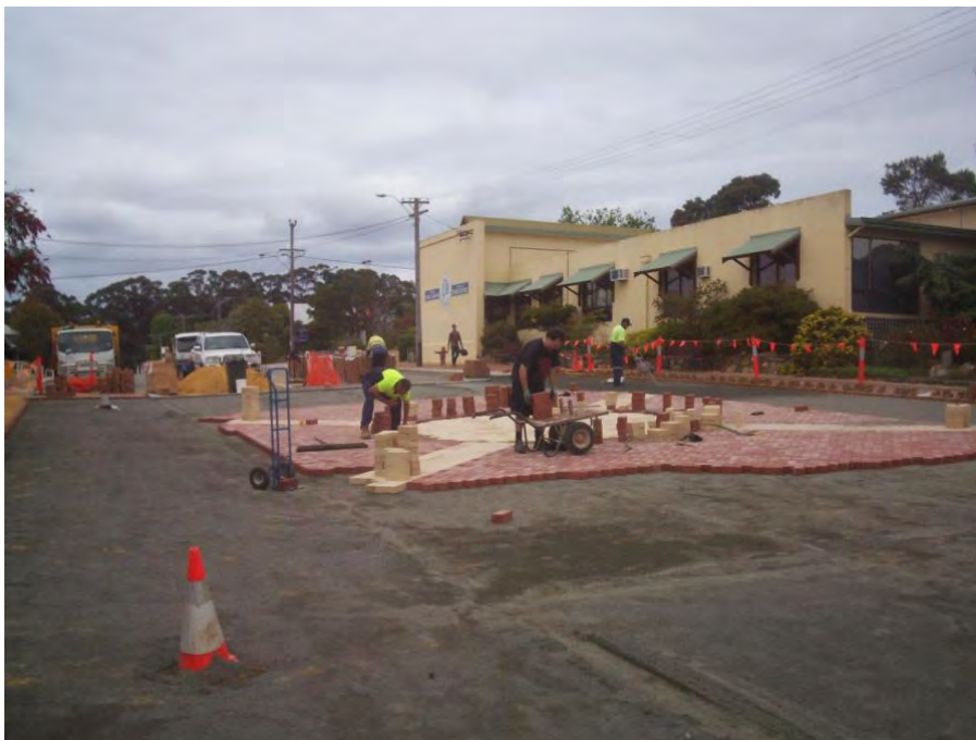
(Paving crew at work on Strickland St Upgrade)
