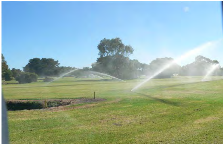
(New reticulation at work on Golf Course)
