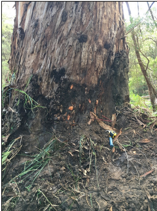
Image 8: Probe location no. 4. The probe was able to be inserted 1000mm into the trunk on the tension side of the trees lean.
