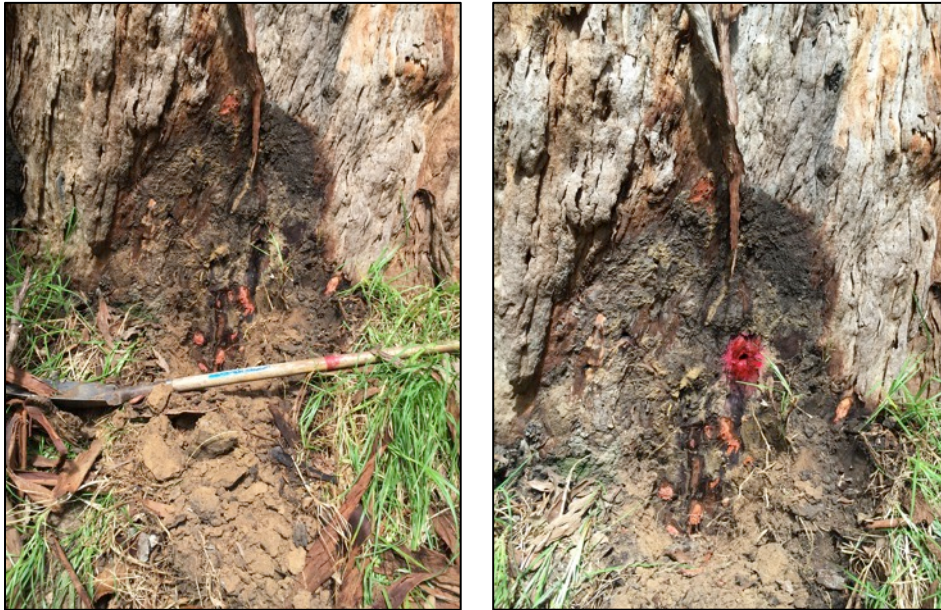
Images 4 & 5: With the termite mud removed the entry-points for the termites were visible.
