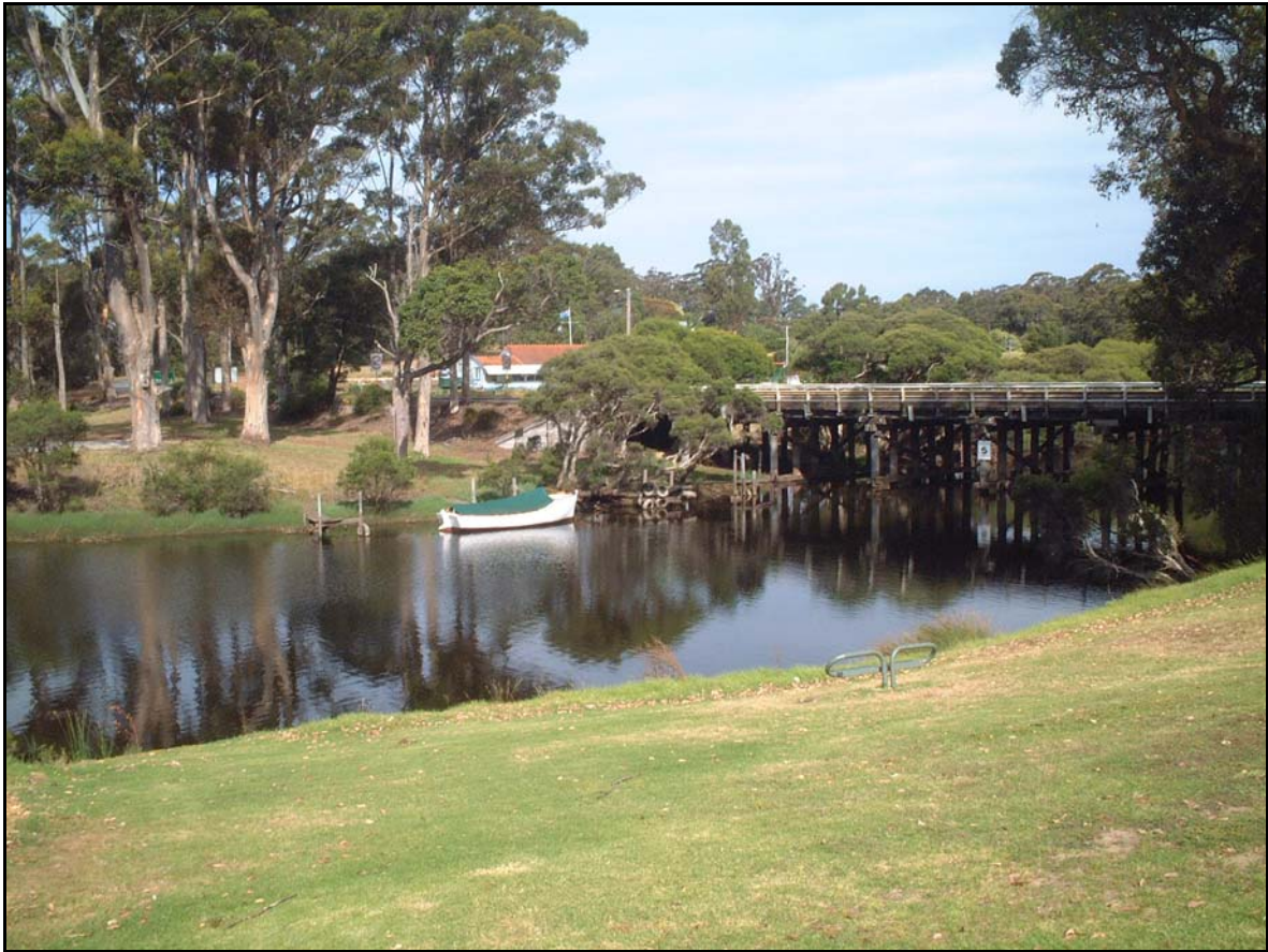
Photo 2. River Zone 1 Looking down river to the road bridge and classic boat mooring area
