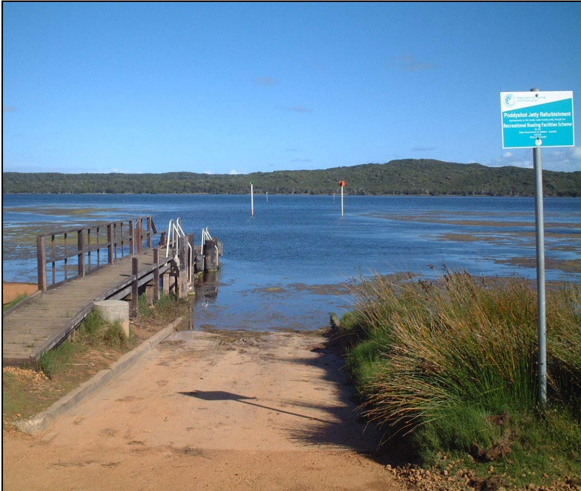
Photo 15. Poddyshot Jetty and Boat Ramp note the narrowness and shallowness of the access ramp
