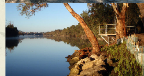
Image 1: Example bank protection works (Photos for illustrative purposes only).
