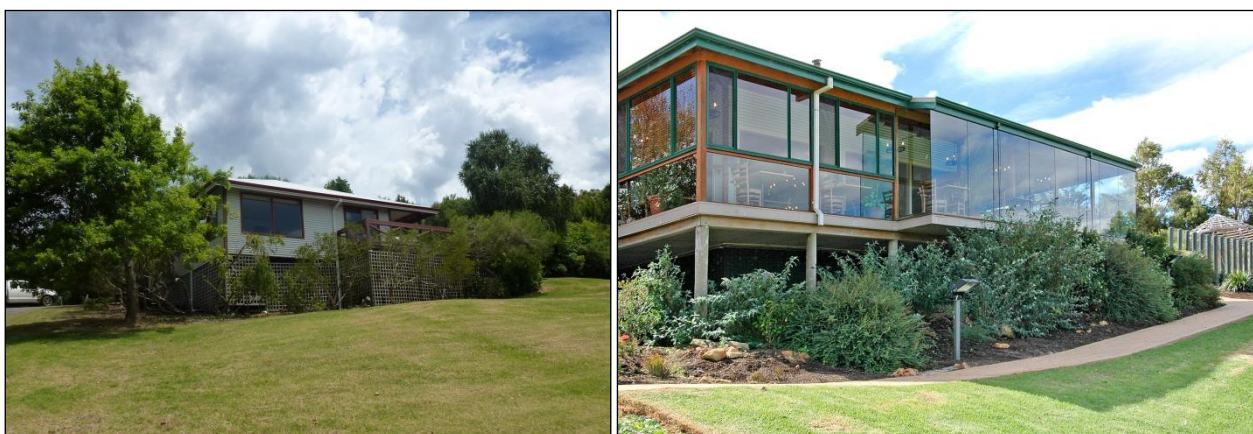
Existing development on-site demonstrating pole construction on a sloping site and screening measures for the underside.
