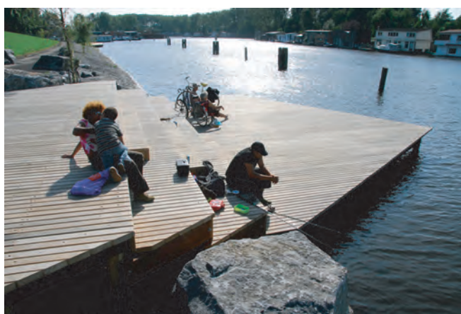
IMAGE: FIXED STEPPED JETTIES WITH COMPOSITE TIMBER DECKING
