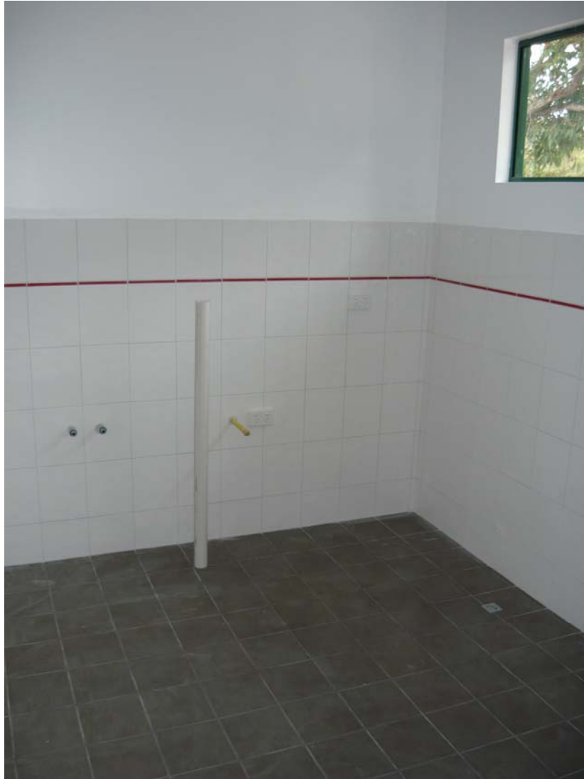
Utility Room – Wall and Floor Tiling, Basin Water Supply and Drainage
