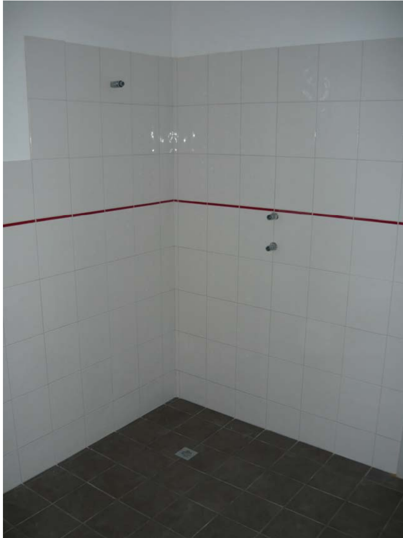
Utility Room – Wall and Floor Tiling, Shower Water Supply and Drainage
