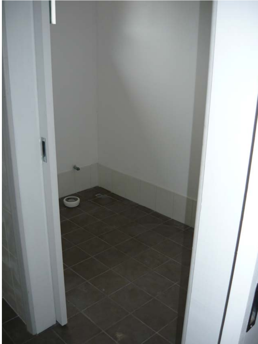
Toilet - Wall and Floor Tiling, Water Supply and Drainage
