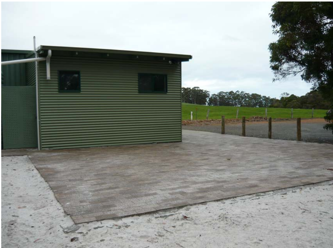
Brick Paving and Metal Door to Screen Gas Bottles
