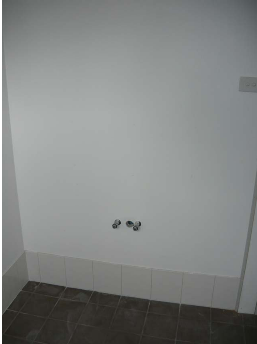
Toilet - Wall and Floor Tiling, Hand Basin Water Supply and Drainage
