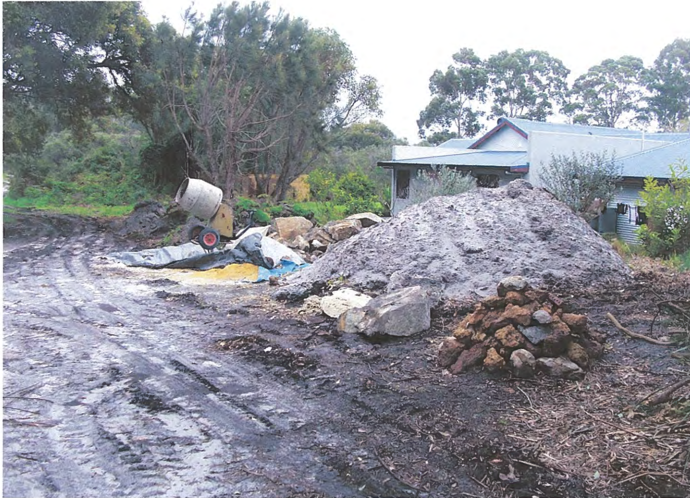
WORK BEING CARRIED OUT IN ROW.
