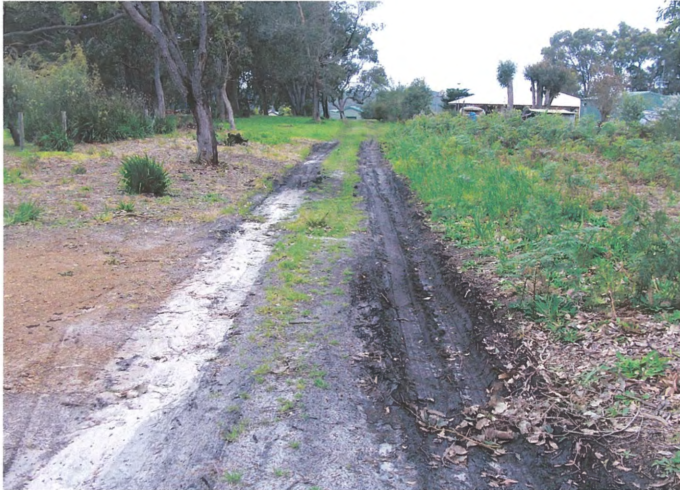
RUTS NEAR ENTRANCE OF ROW 9 PARK BOUNDARY
