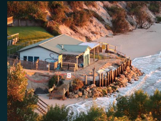
Timber retaining wall, and rock scour protection
