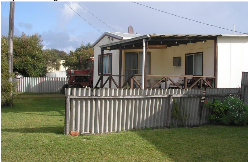
Property to the west. Small verandah existing.
