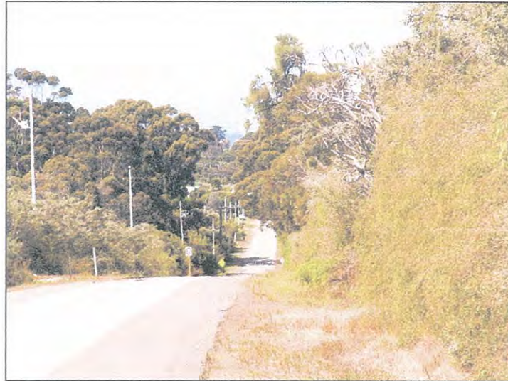
Figure 15- Constructed and sealed Lights Road and Overhead Power Supply
