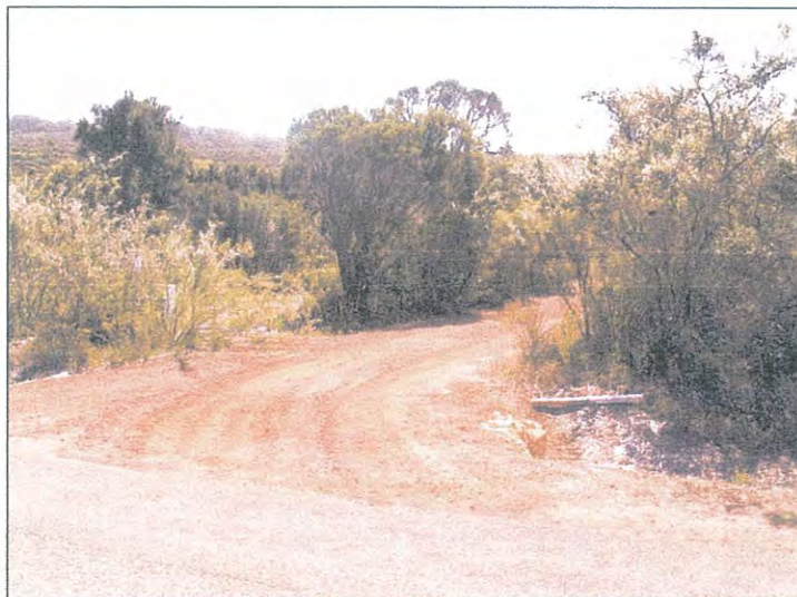
Figure 12- Access to Lot 93 from Lights Road
