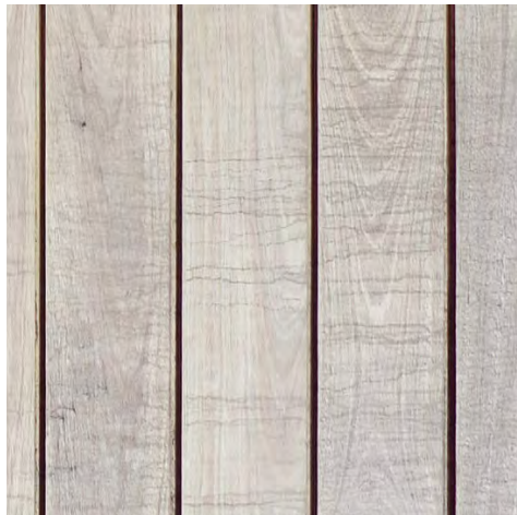
Weathered timber battens & screens
