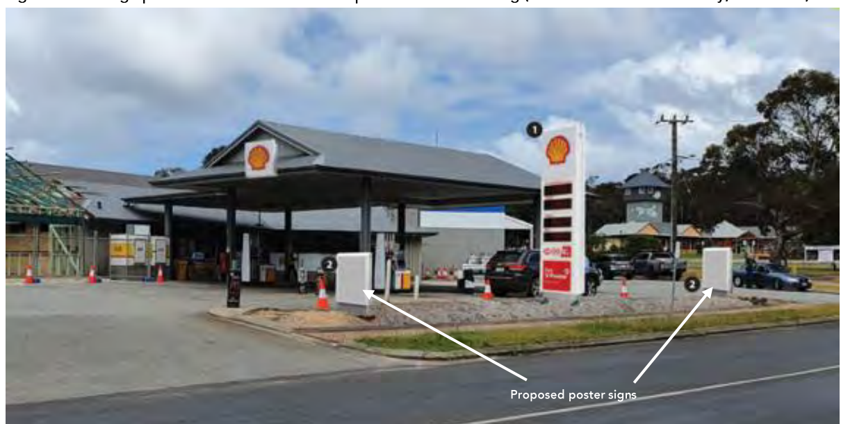
Figure 2 – Photograph of Service Station Redevelopment and Re-Branding (taken from South Coast Hwy, Nov. 2020)
