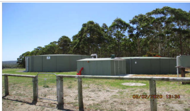
Water tanks for DFES
