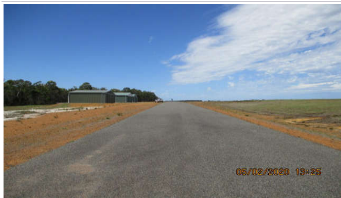
Established portion of second vehicle access road to subject sites
