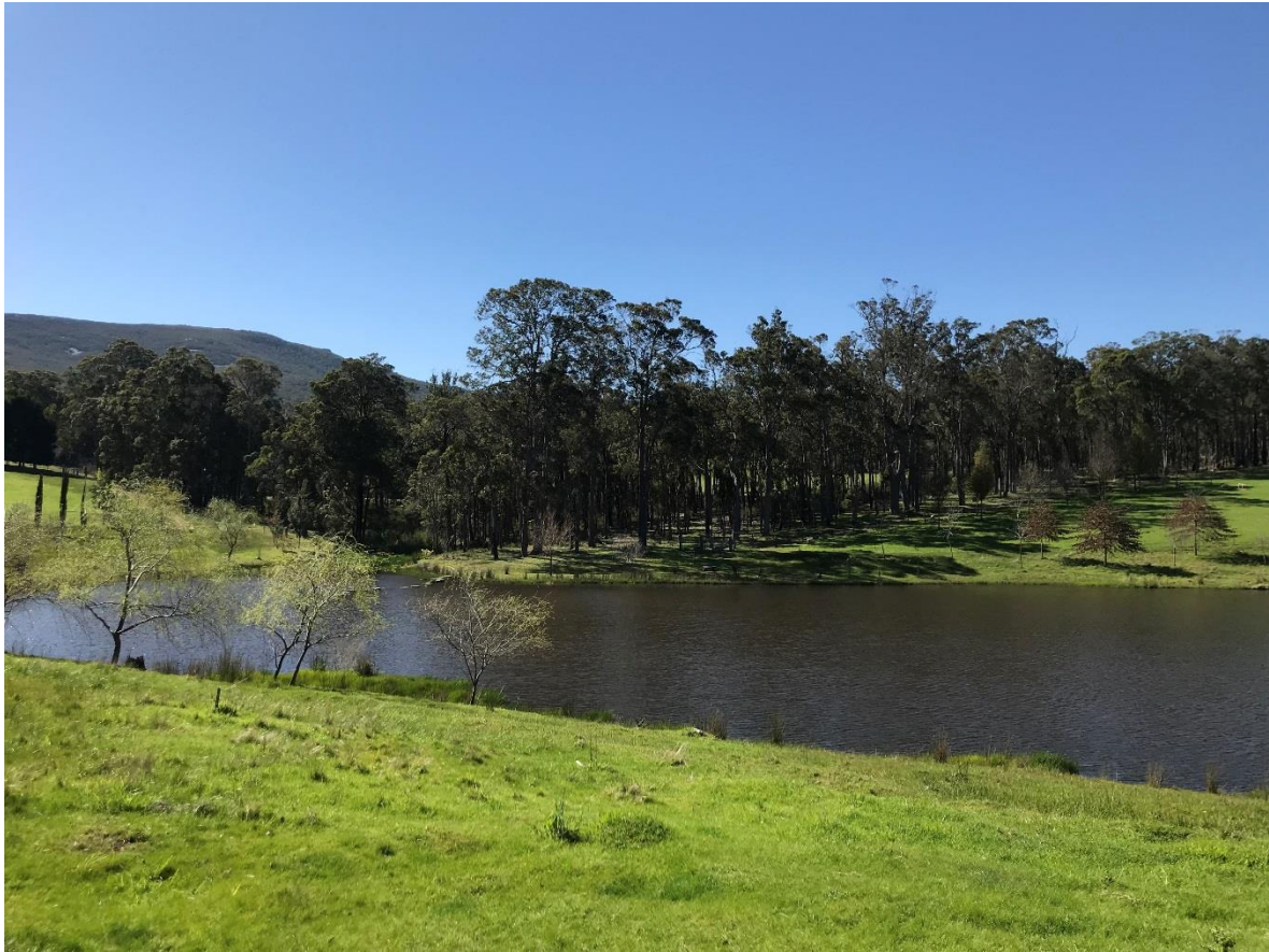
Large gully dam
