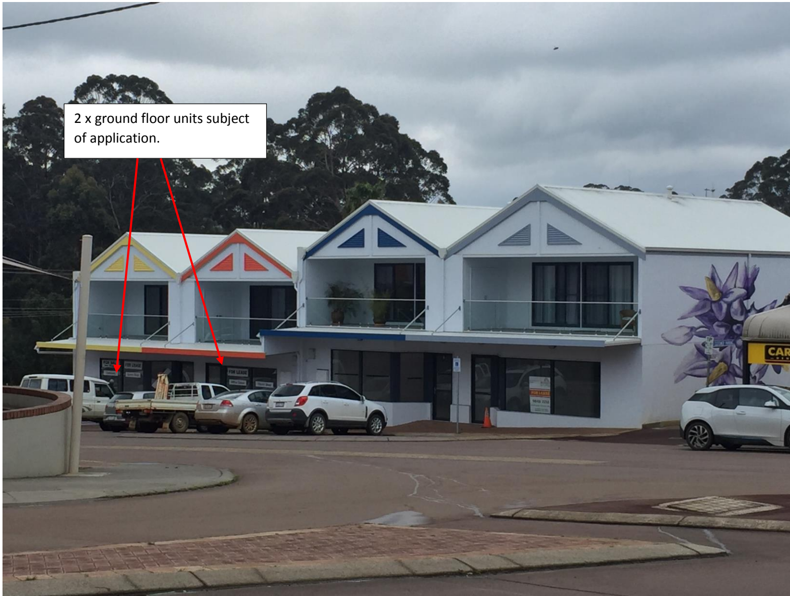
Streetscape photo - No.1/3A (Strata Lot 2/ Lot 102) and No.3/3A (Strata Lot 1/ Lot 102) Strickland Street, Denmark
