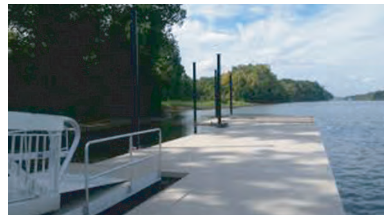
IMAGE: FLOATING JETTY
