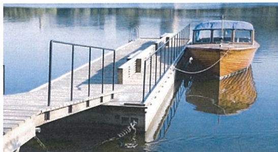
IMAGE: FLOATING JETTY WITH COMPOSITE TIMBER DECKING
