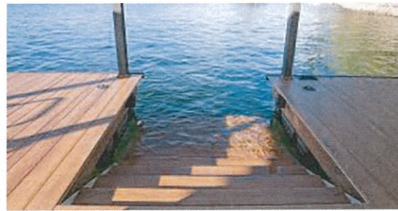
IMAGE: WATER ACCESSIBLE STEPPED JETTIES WITH COMPOSITE TIMBER DECKING
