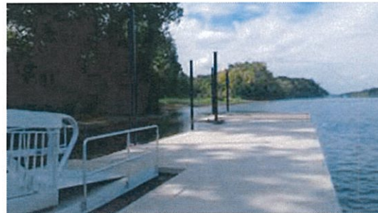
IMAGE: FLOATING JETTY
