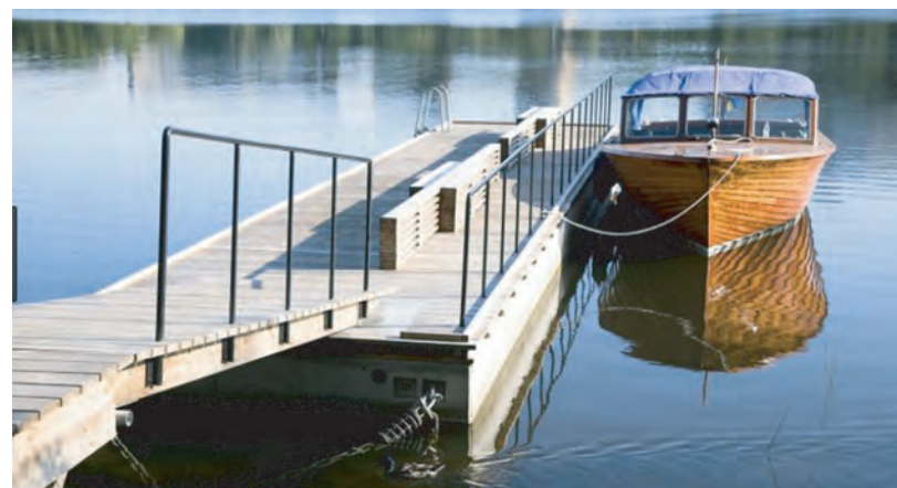
IMAGE: FLOATING JETTY WITH COMPOSITE TIMBER DECKING
