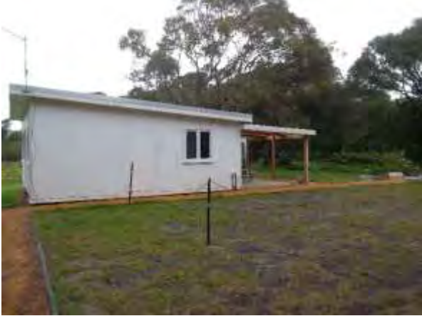
Photograph 1 – View of the existing house north central of the Subject Site.
