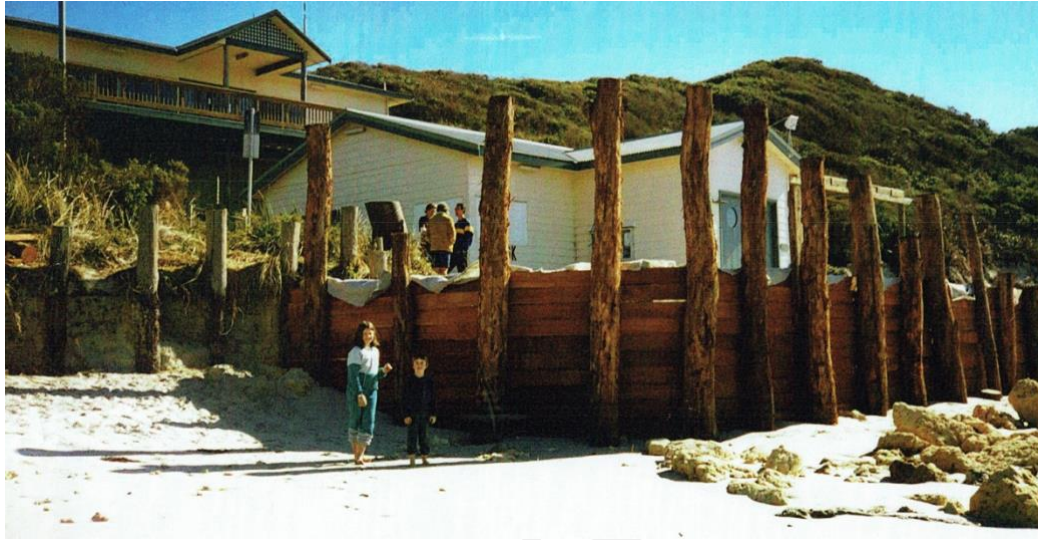
Figure 5.3 Timber Retaining Wall in front of the Ocean Beach SLSC Buildings (date unknown, courtesy of the Denmark SLSC)
