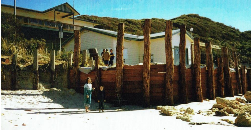
Figure 5.3 Timber Retaining Wall in front of the Ocean Beach SLSC Buildings (date unknown, courtesy of the Denmark SLSC)
