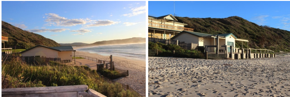
Figure 2: Ocean Beach During Reconnaissance Site Inspection (June 2016)
