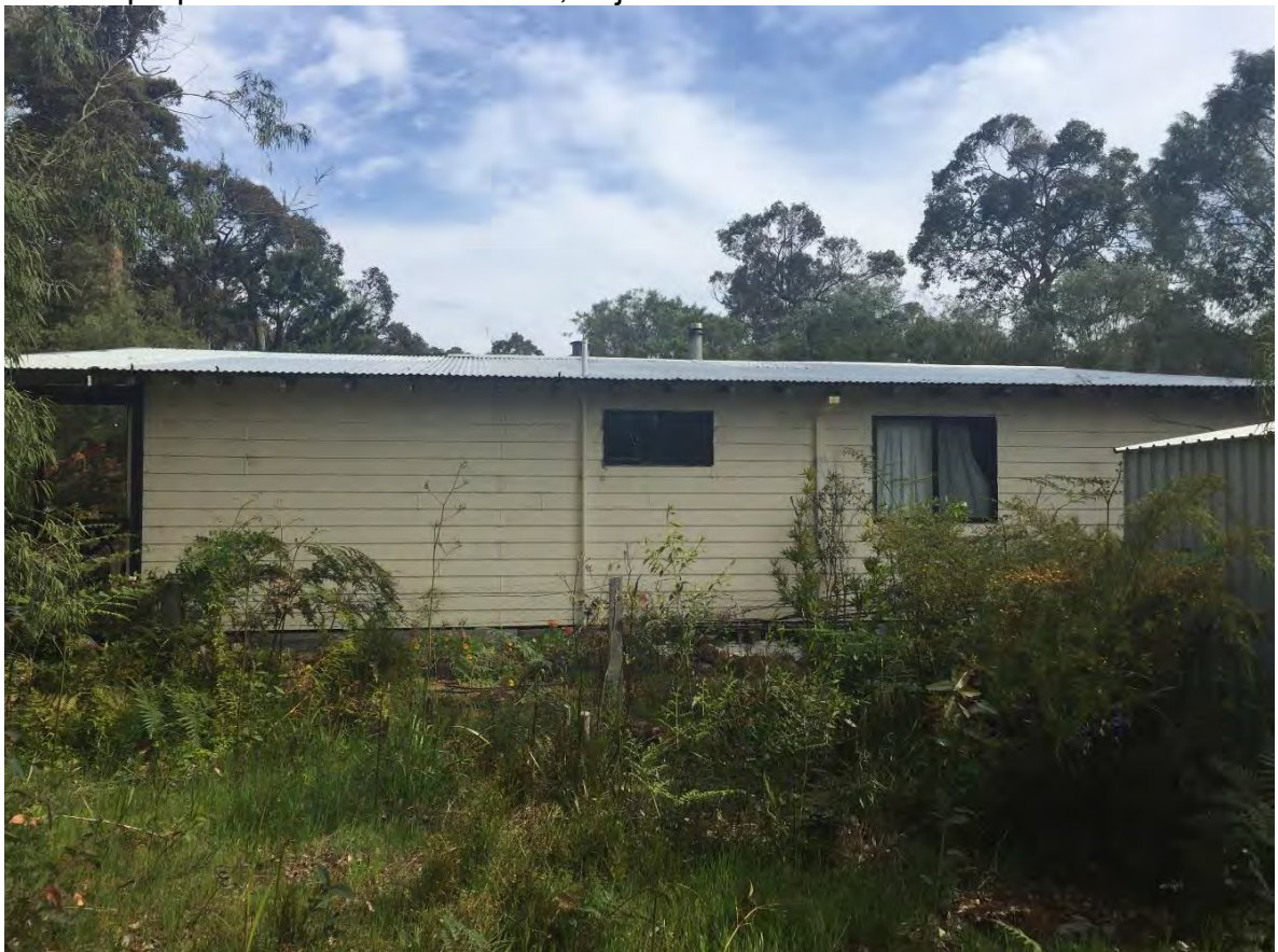
Side view of adjoining residence (No.115 Inlet Drive)
