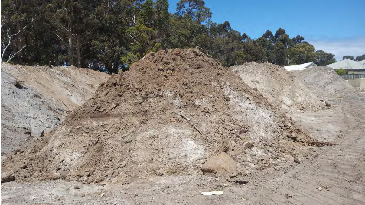
Clay soil that is unsuitable for foundation material
