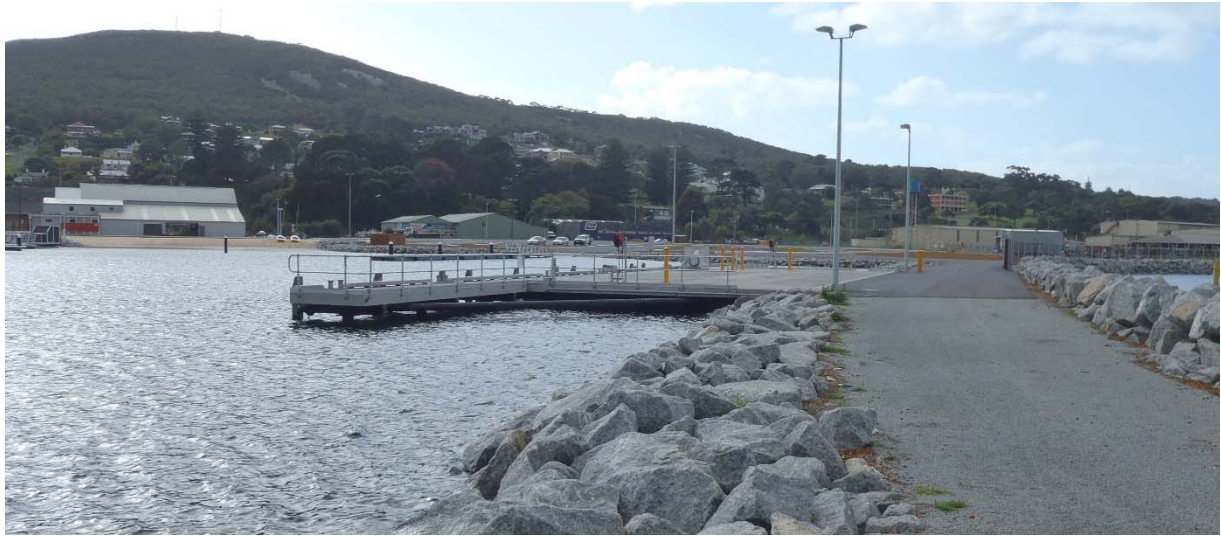
Figure 4.6 Example of Wharf
