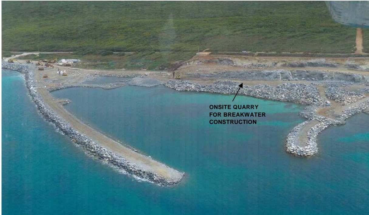
Figure 4.11 Augusta Boat Harbour Construction
