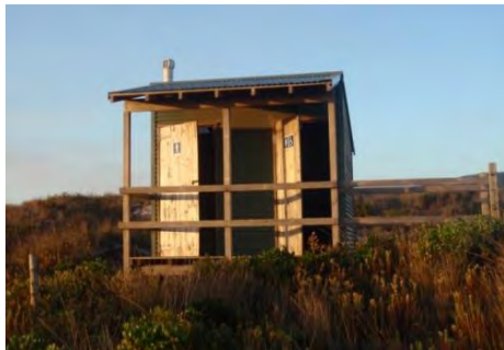
Composting toilets at Lights Beach
