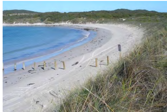
Vehicle access bollards closure at Peaceful Bay allowing access for emergency vehicles only
