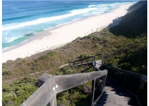
Pedestrian access timber staircase at Back Beach
