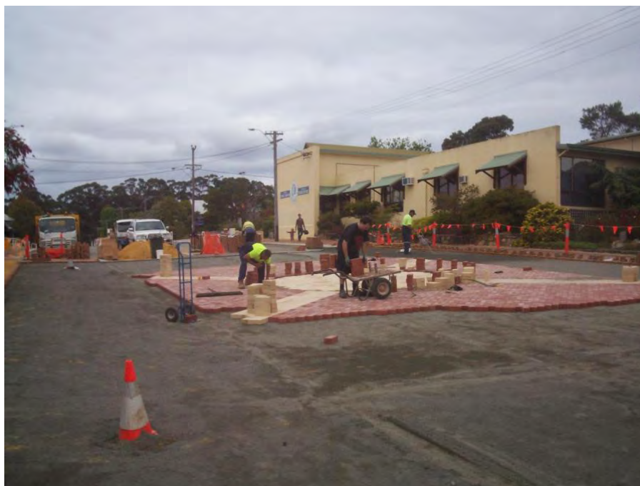
(Paving crew at work on Strickland St Upgrade)
