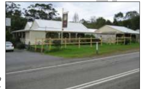
FIG 2.3: Typical streetscape characteristics within Nornalup.
