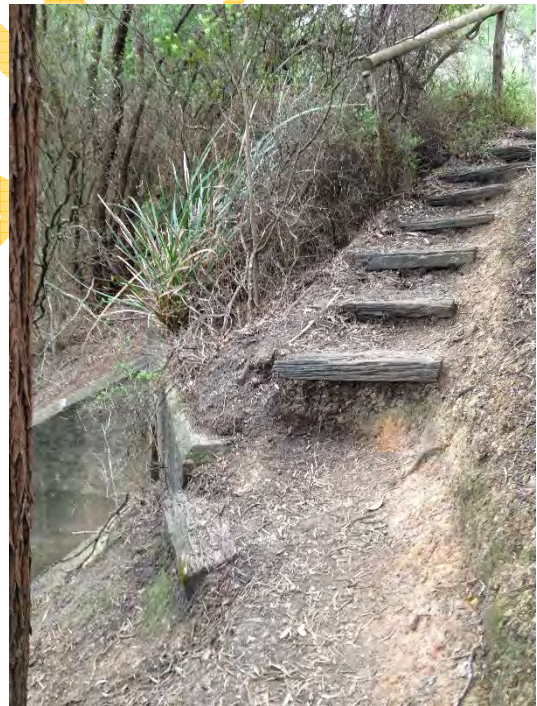
Plate 12 Access to the Springdale Tunnel to the south of the Heritage Trail requires upgrade of steps and handrail
