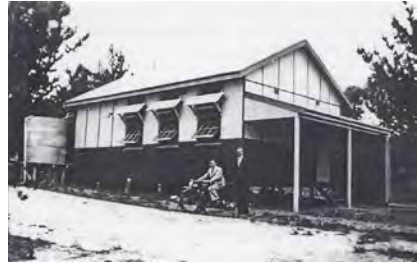
IMAGE 02: CARMARTHEN SCHOOL IN SITU 1940
