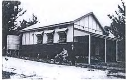
IMAGE 02: CARMARTHEN SCHOOL IN SITU 1940
