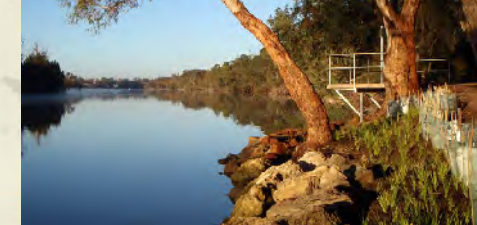
Image 1: Example bank protection works (Photos for illustrative purposes only).
