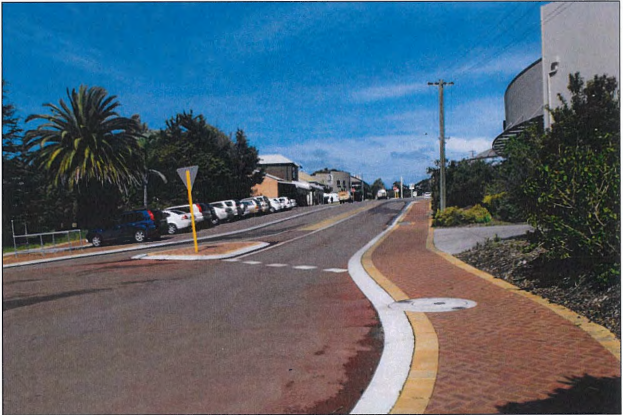
Right angle car parking located adjacent to Lot 200
