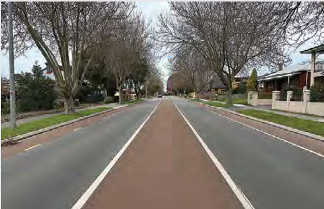
Middleton Road cycle path Credit: City of Albany
