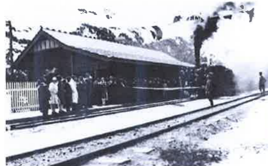
DENMARK RAILWAY STATION
