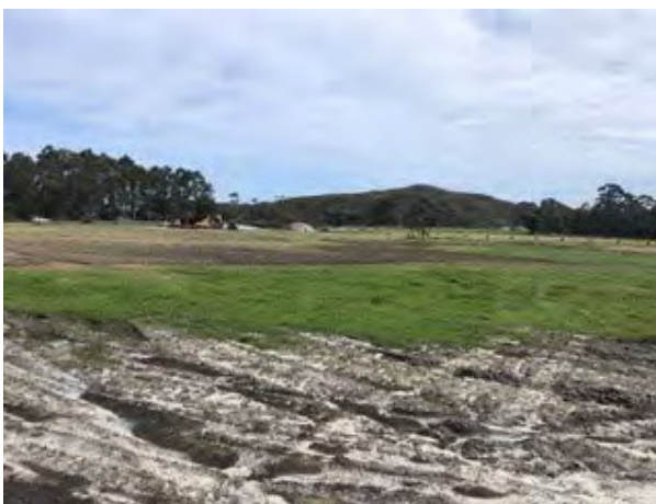
Figure 5: Bottom of dam looking SW
