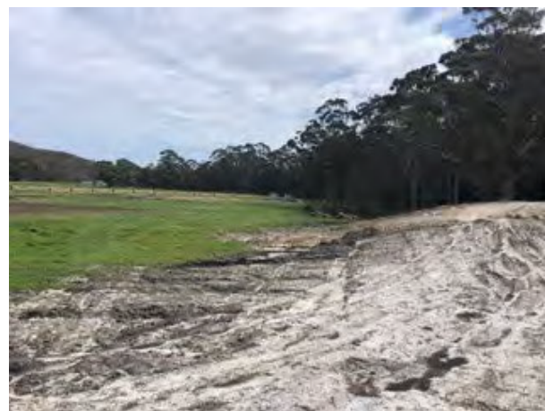
Figure 6: Bottom of dam looking W
