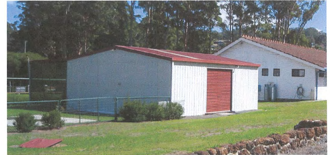
View 02: Existing shed - View from SOUTH EAST
