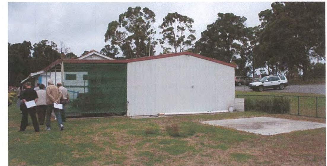
View 04: Existing shed - View from SOUTH WEST
